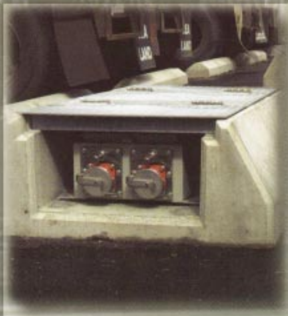
4-Gang Bunker Mount Assembly (2 other side) Cat. No. E4-R32-480-30-22SB-SP-220285 Port of Tacoma
